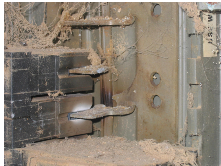
Photo 5: 15 year old panel with a 170 °F (77°C) hot spot.
