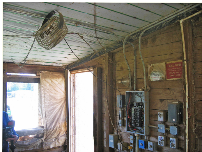
Photo 1: Electrical panels with covers removed and fans blowing on the breakers to keep them cool – sure signs of an inadequate electrical system that is likely to fail abruptly.
